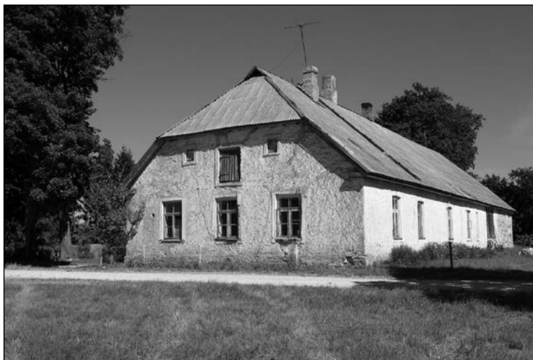
3: Endine Esna vallakool Kareda külas. 1867. a ehitatud koolimaja oli rehielamu, milles asusid nii klassiruumid kui ka rehetuba ja -alune. Foto M. Tamjärv, 2006. 3: Former Esna parish school in Kareda village. The schoolhouse built in 1867 was a barn-dwelling housing both classrooms and the threshing floor and kiln room. Photo by M. Tamjärv, 2006.
